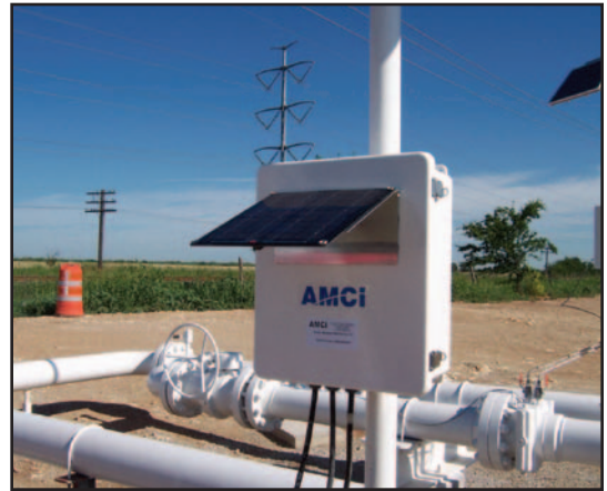
■ (Left) The Satellite Monitoring Unit (SMU) illustrated above includes a SatAlarm Interface Device (SID), satellite modem, terminal blocks and a backup lithium battery. (Right) This pole-mounted unit is equipped with American Millennium Corporation Inc.'s (AMCi's) integrated solar panel power supply.
